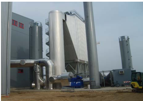
Dry sorption with high temperature electrostatic precipitator and NO x catalyzer
