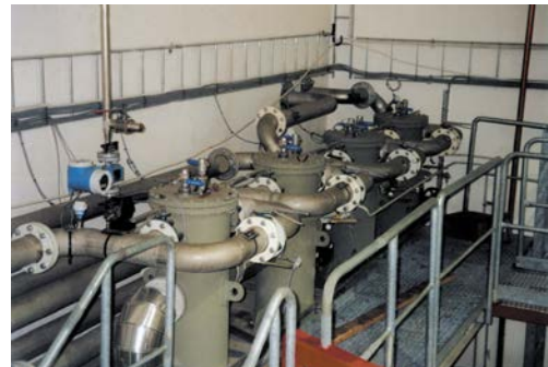
Simple inspection and maintenance of the heat exchangers due to pre-chambers
